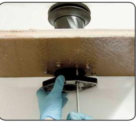
2. Tighten six M6 precote coated screws (~8 Nm/ 70 in-lb)
